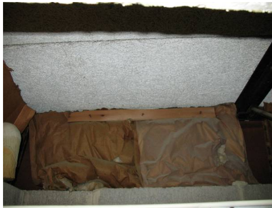
View of exterior wall and ceiling insulation from plenum
