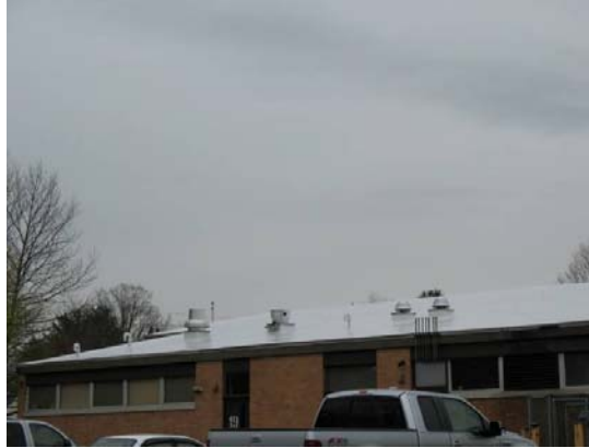
2 year old White rubber membrane roof
