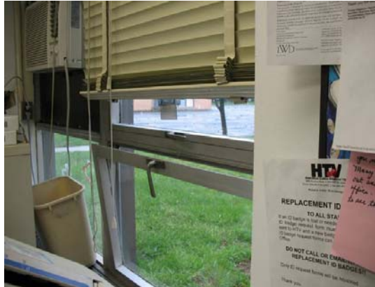
Single pane window located in main office
