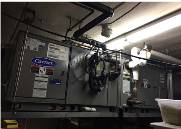
Image 9: AHU and Electric Resistance Heater
