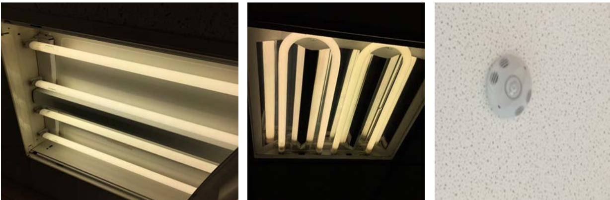
Image 4: Fluorescent T8 and Ceiling Mounted Sensors
