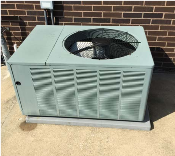
Image 6: 3 Ton Rheem Split AC & Thermostat
