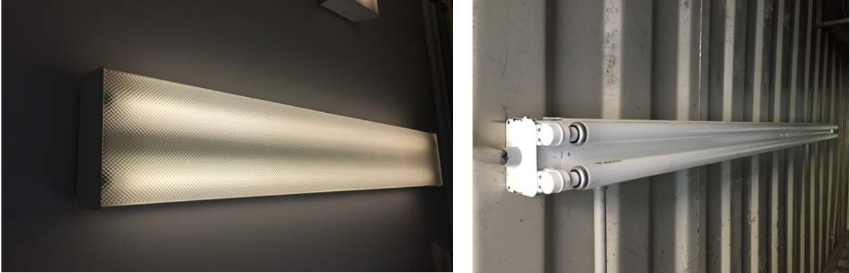
Image 3: Fluorescent T8 & T12 Fixtures
