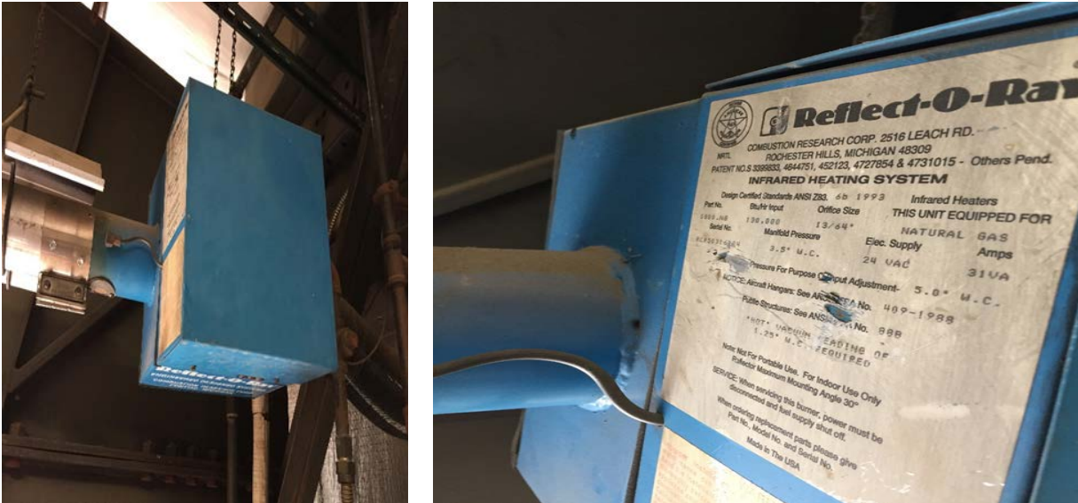
Image 8: Suspended Radian Gas Heaters
