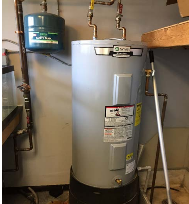
Image 5: Domestic Hot water
