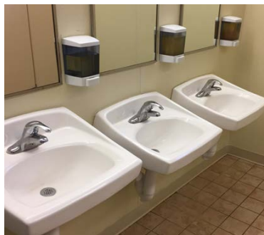
Image 8: Typical Restroom Faucets
