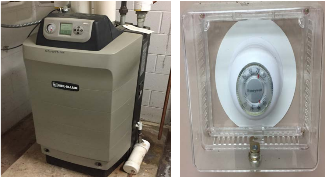
Image 5: Heating Hot Water System
