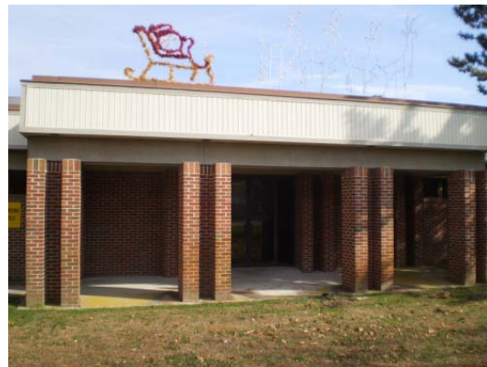
Partial East Façade
