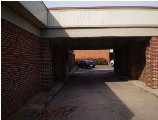
Partial South Façade
