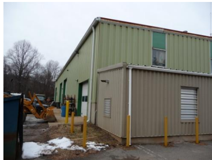
Rear and Left Side Façade
