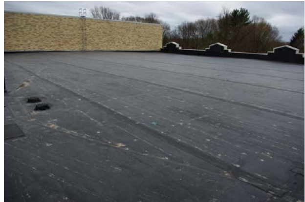
Flat Area of High School Roof
