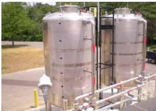
The gas conditioning equipment includes hydrogen sulfide removal through the use of H<sub>2</sub>S scrubbers.
