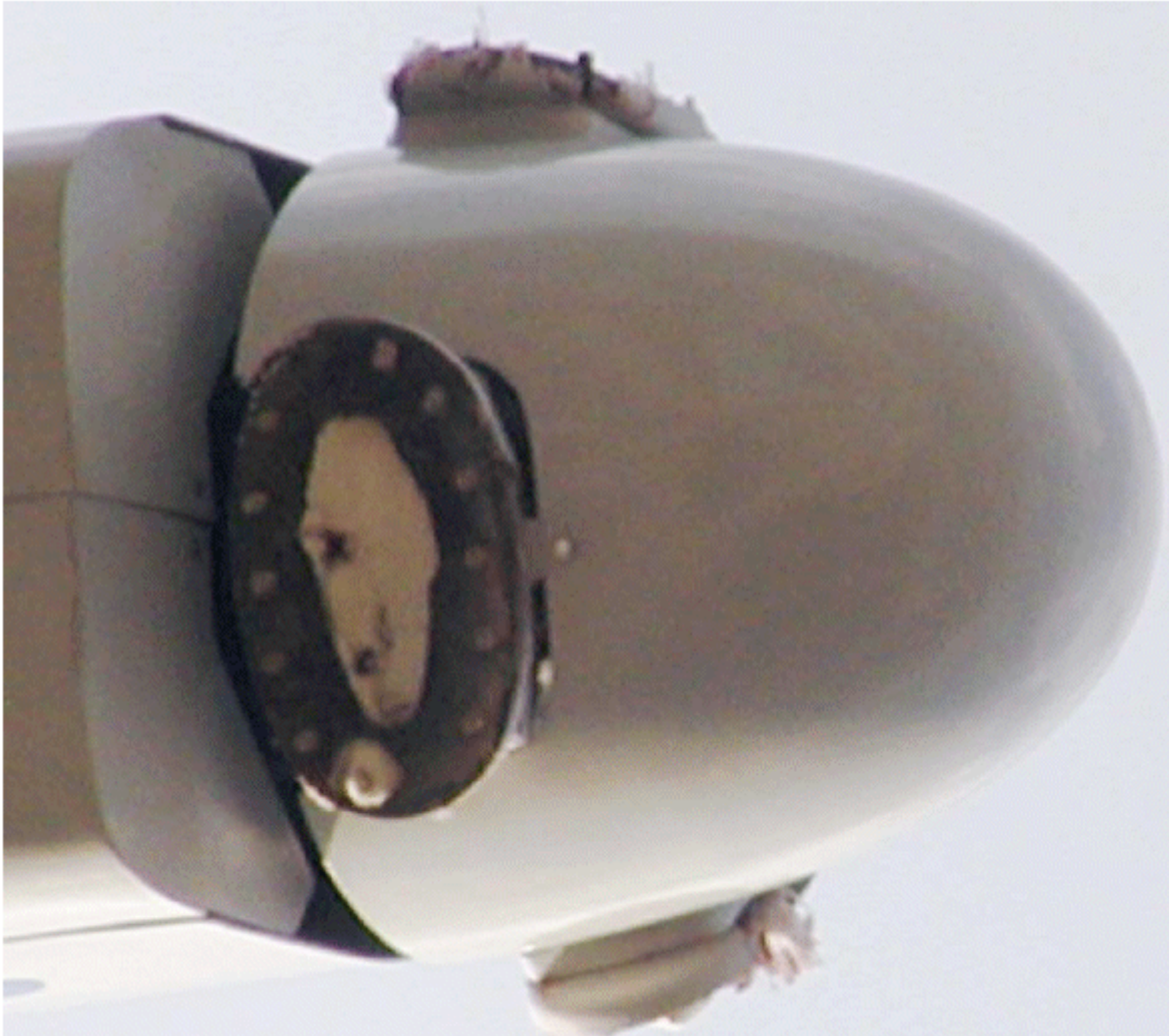
Figure 1. The Knoeller site turbine hub after the blades had separated
