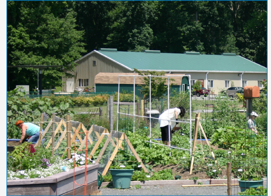
Middlesex County's Agricultural Extension building provides office space for the EARTH Center in Davidson's Mill Pond Park (pictured above). Energy efficiency improvements reduced monthly utility expenses by half.
