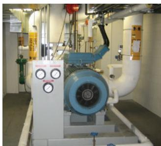
A steam-driven back pressure turbine provides 550 kW of electrical power and low pressure steam for use in the pharmaceuticals research process.
