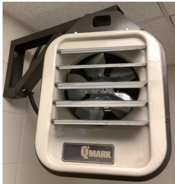
Electric Resistance Heaters
