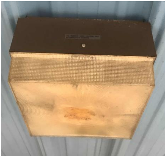
Exterior HPS Fixture
