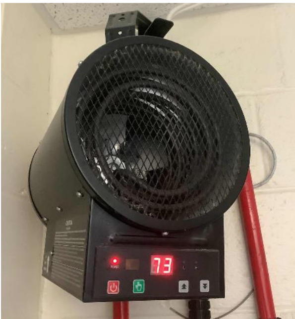
Electric Resistance Heaters
