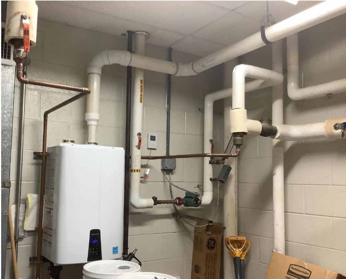
Water Heater and Circulation Pump
