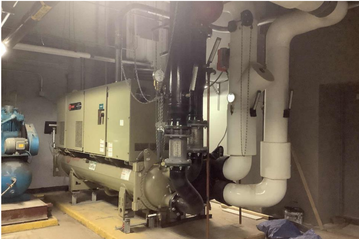
Water-cooled Chiller
