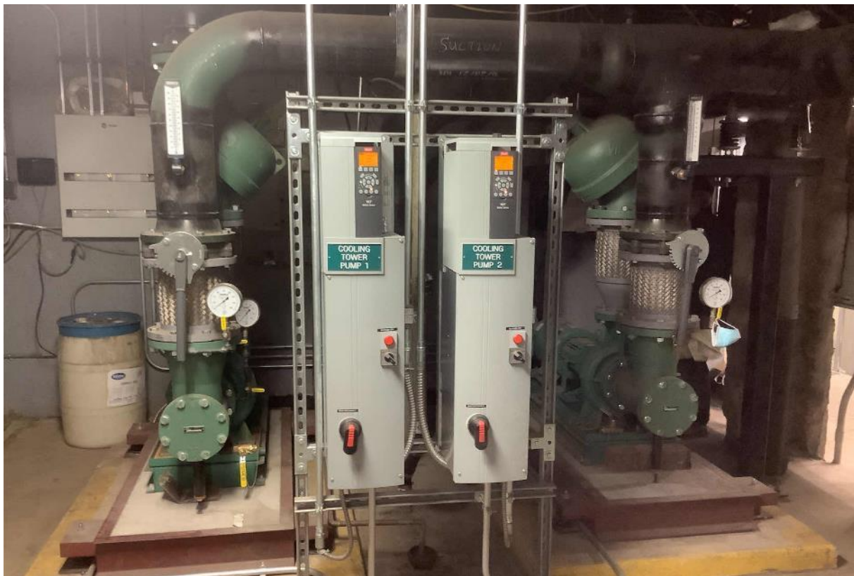
Condenser Water Pumps
