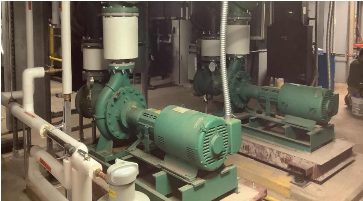
Heating Hot Water Pumps
