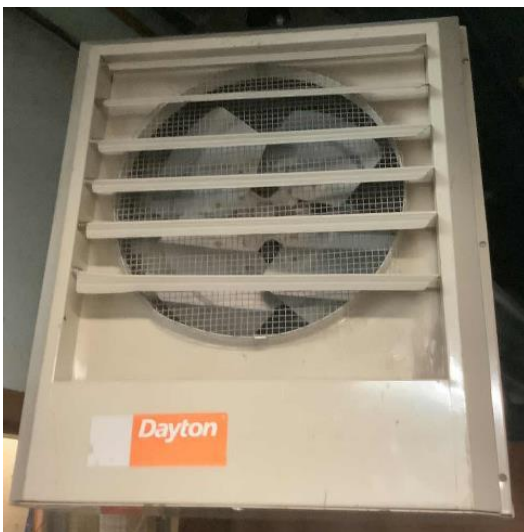
Electric Resistance Heaters
