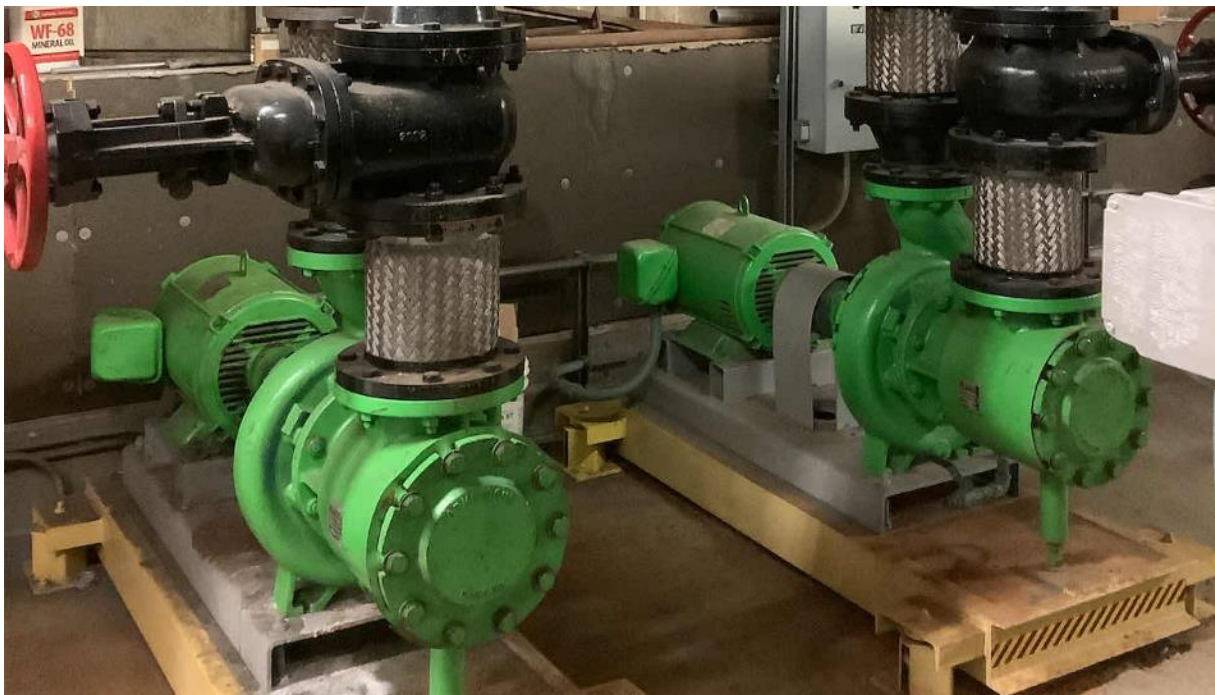
Condenser Water Pumps
