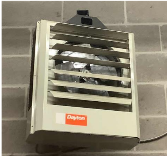
Electric Resistance Heaters
