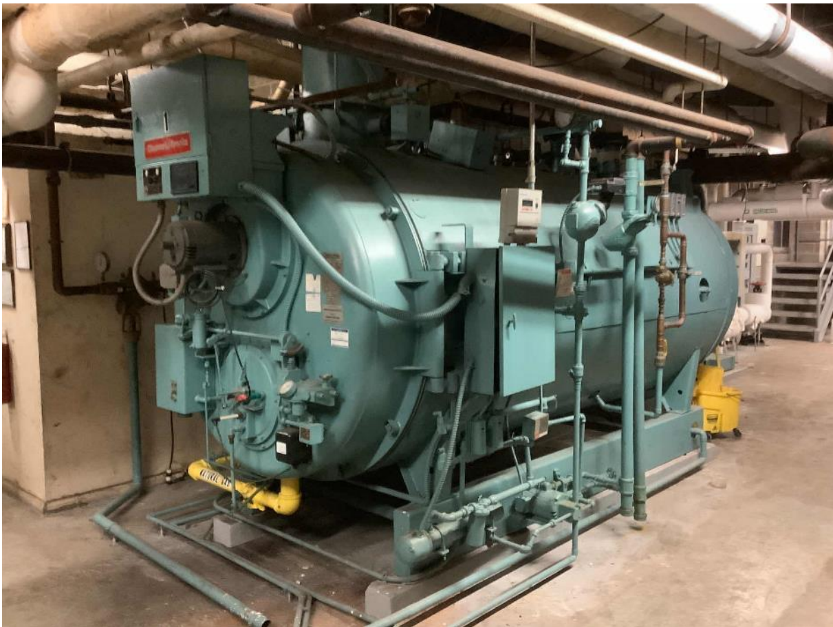
Hot Water Boiler
