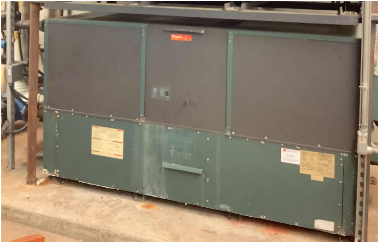
Hot Water Boiler
