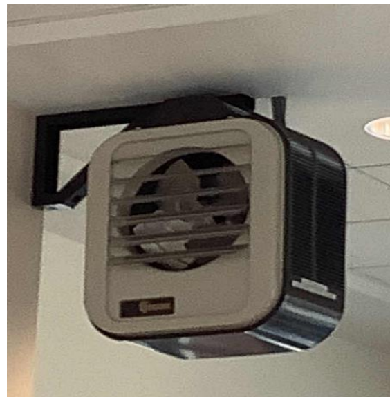
Electric Resistance Heaters
