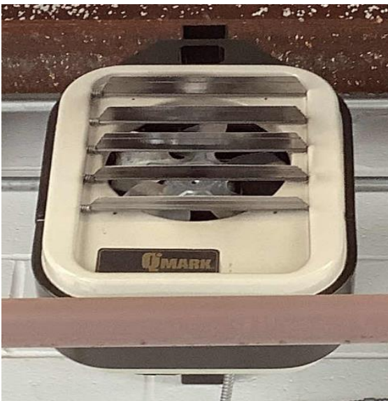
Electric Resistance Heaters
