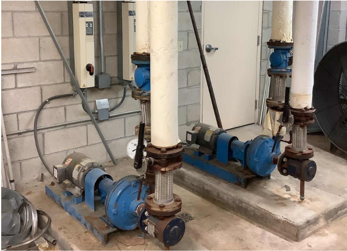
Heating Hot Water Pumps
