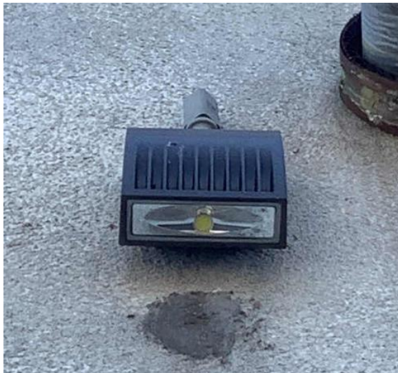
Exterior LED Fixture
