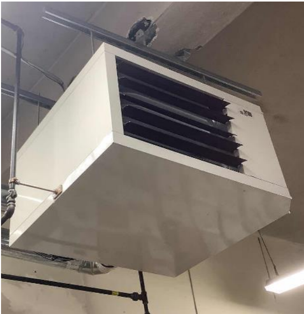
Gas-fired Unit Heaters
