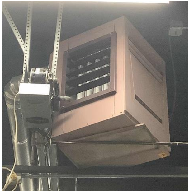
Gas-fired Unit Heaters
