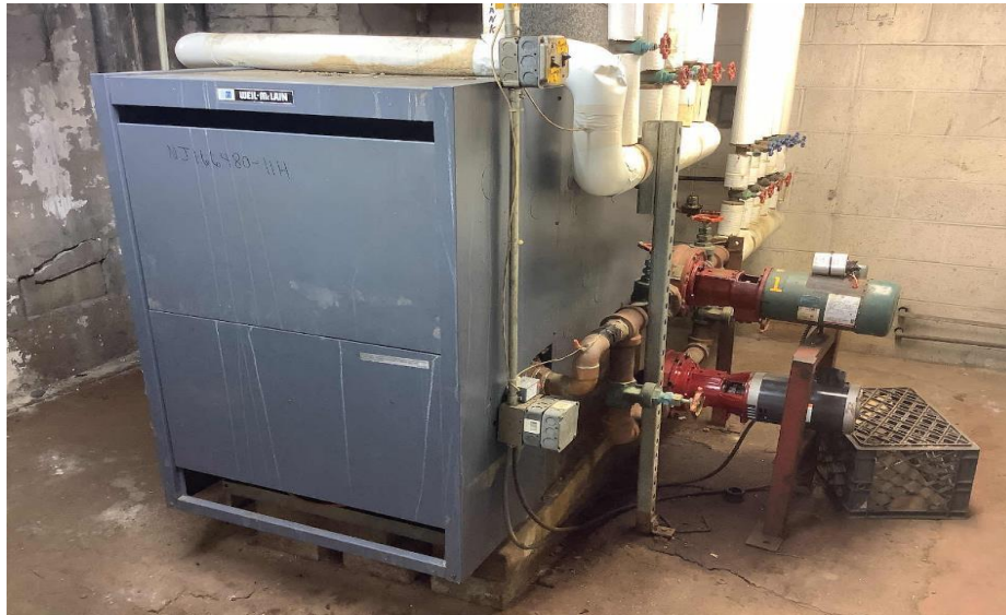
Hot Water Boiler
