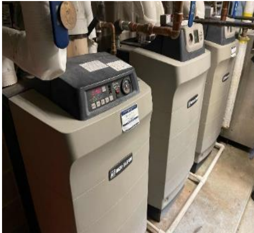
Weil-McLane Condensing Boilers
