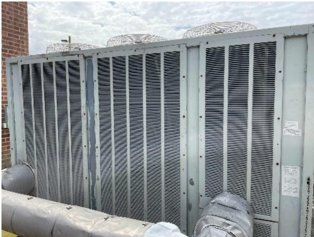
70-ton Air-cooled Chiller
