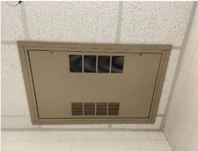
Restroom HW Fan Coil
