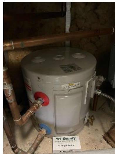
6-gallon Storage Hot Water Heater
