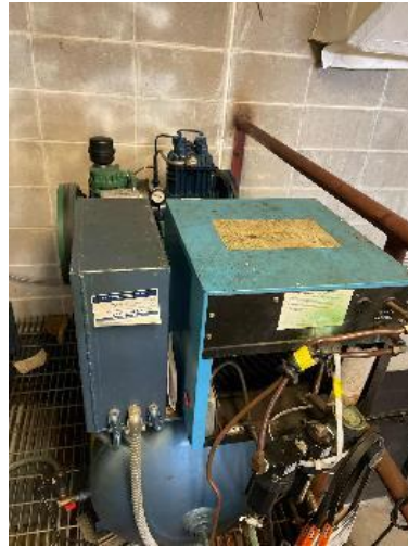
Air Compressor with Refrigerant Desiccant Dryer
