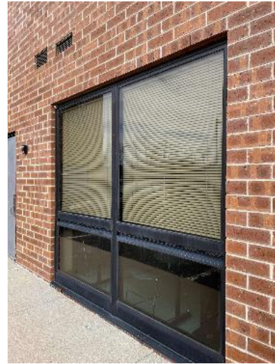
Typical Window Assembly in Brick Façade.
