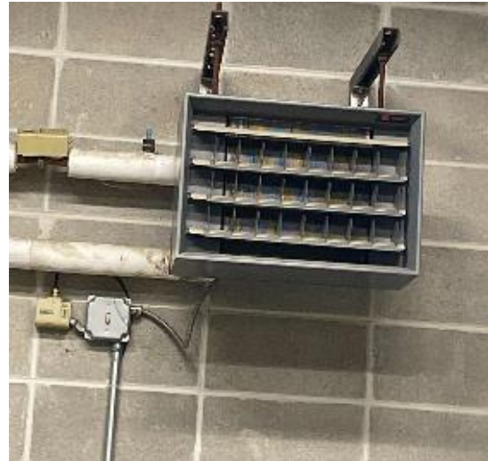
Mechanical Room HW Fan Coil with Pneumatic Thermostat
