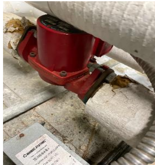
92-Watt Coil Circulator
