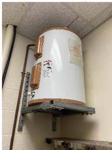
30-gallon Storage Hot Water Heater
