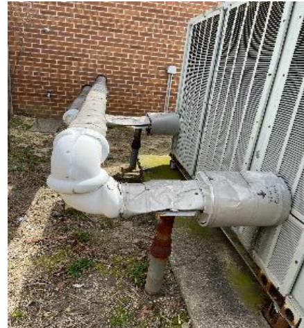
Chilled Water Pipe Insulation
