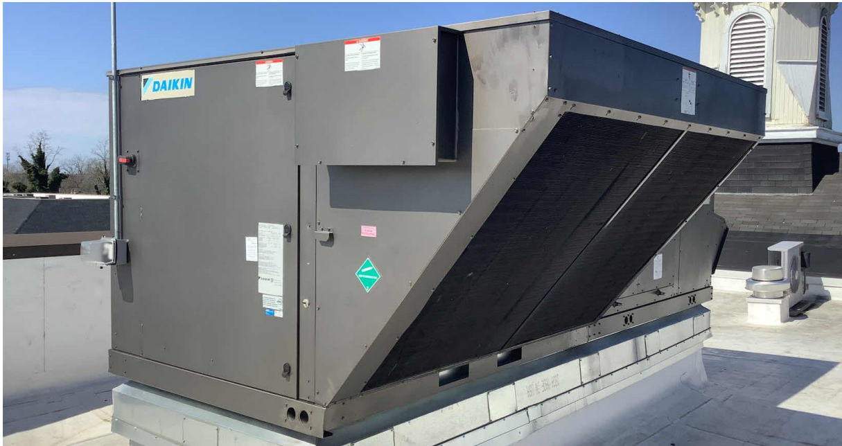
Packaged Air-Source HP Unit
