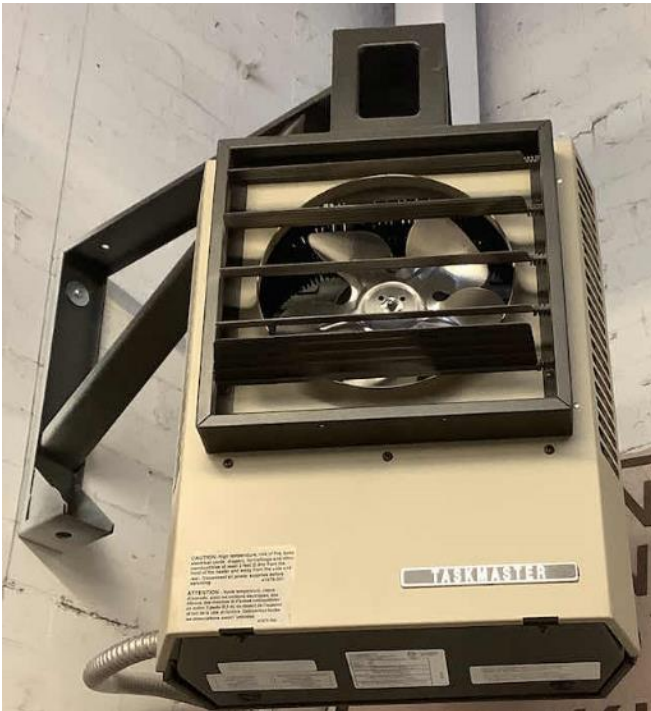
Electric Resistance Heater
