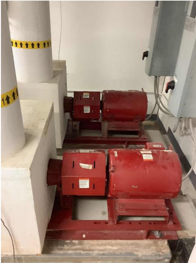
Heating Hot Water Pumps
