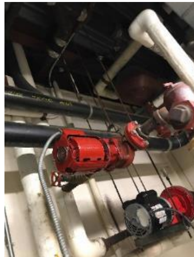
Heating Hot Water Circulating Pumps
