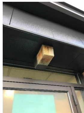
Wall Pack Mount on Roof Overhang
