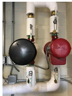
Hot Water Heating Circulator Pumps
