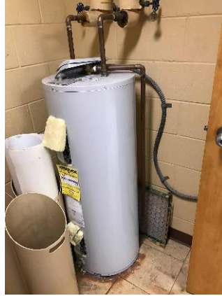
Electric 40-gallon Water Heater.
