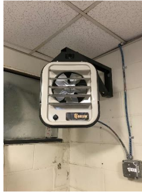
Electric Fan Coil Unit
