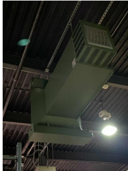
Typical Air Filtration Unit
