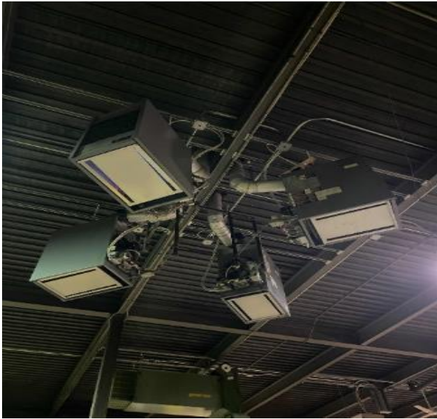
Warehouse Gas-fired Unit Heaters
