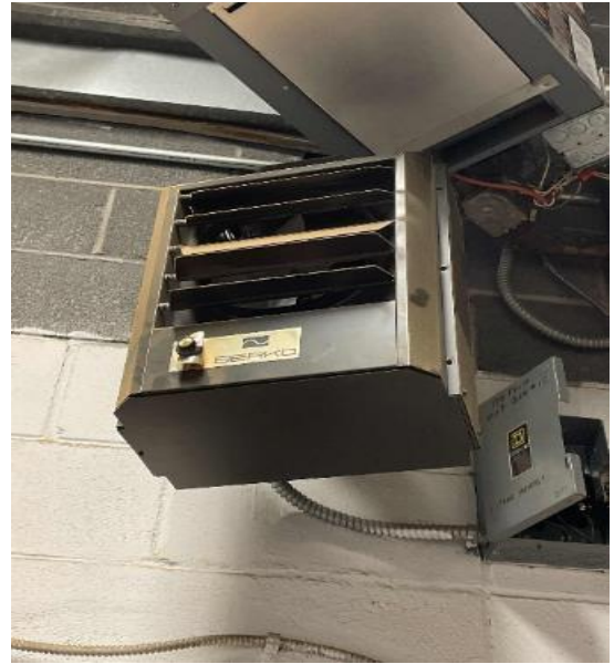
Warehouse Electric Resistance Heater
