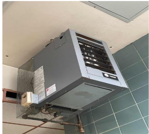
Office Gas-fired Unit Heater
