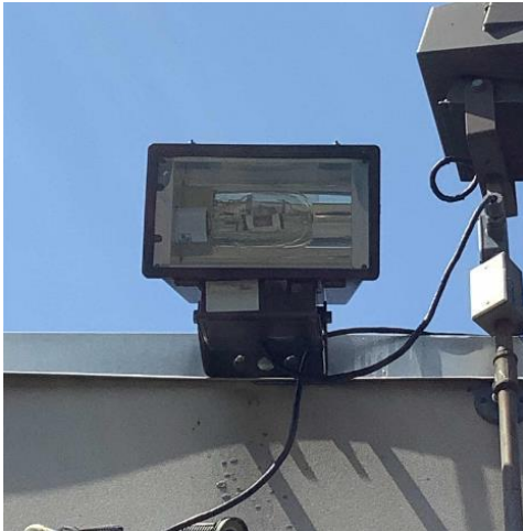
Exterior MH Fixture
