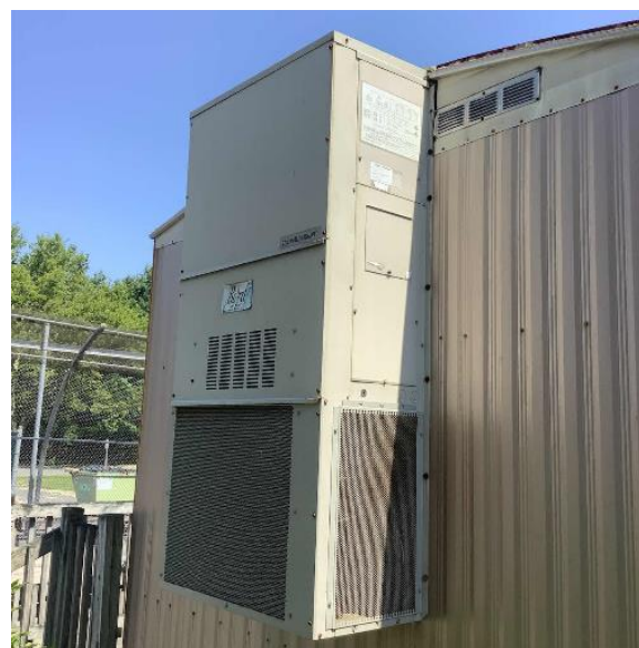
Through-the-Wall AC Unit
