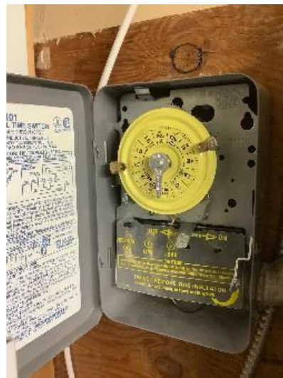
Timer for Front of Building Lights
