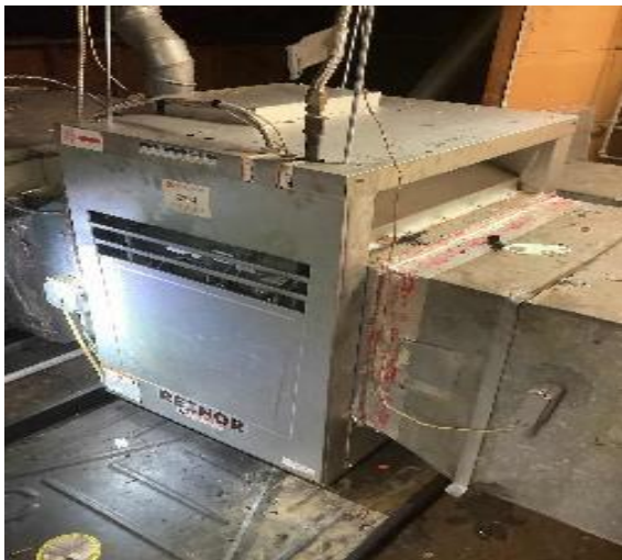
Propane Forced Air Furnace
