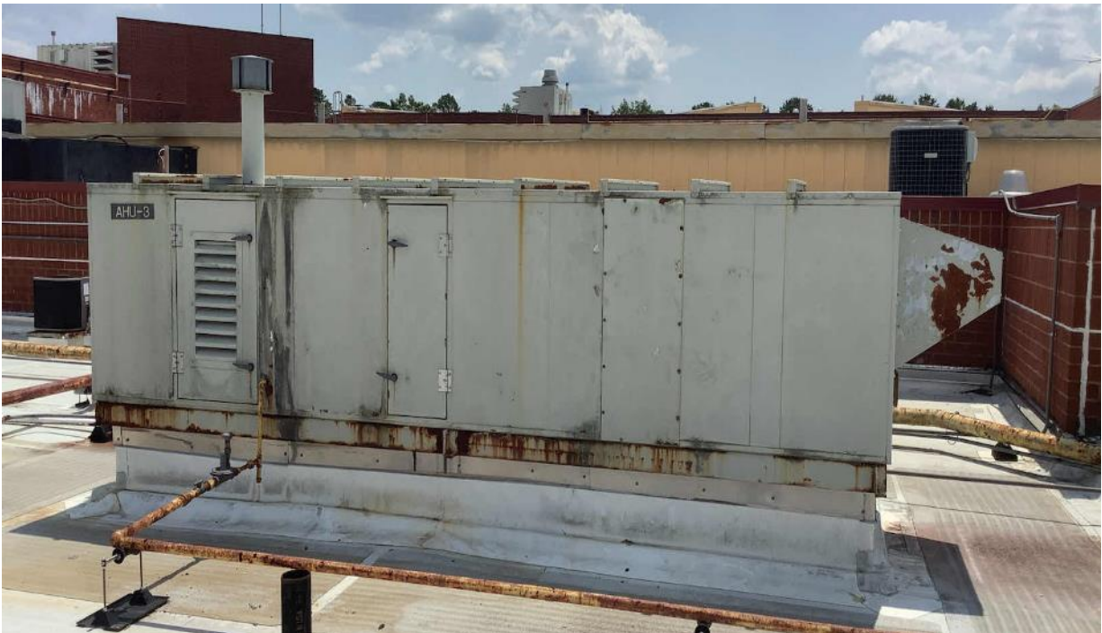
Packaged Unit – Main Building
