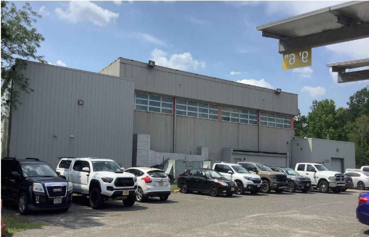
Prosecutors / Records Storage Building
