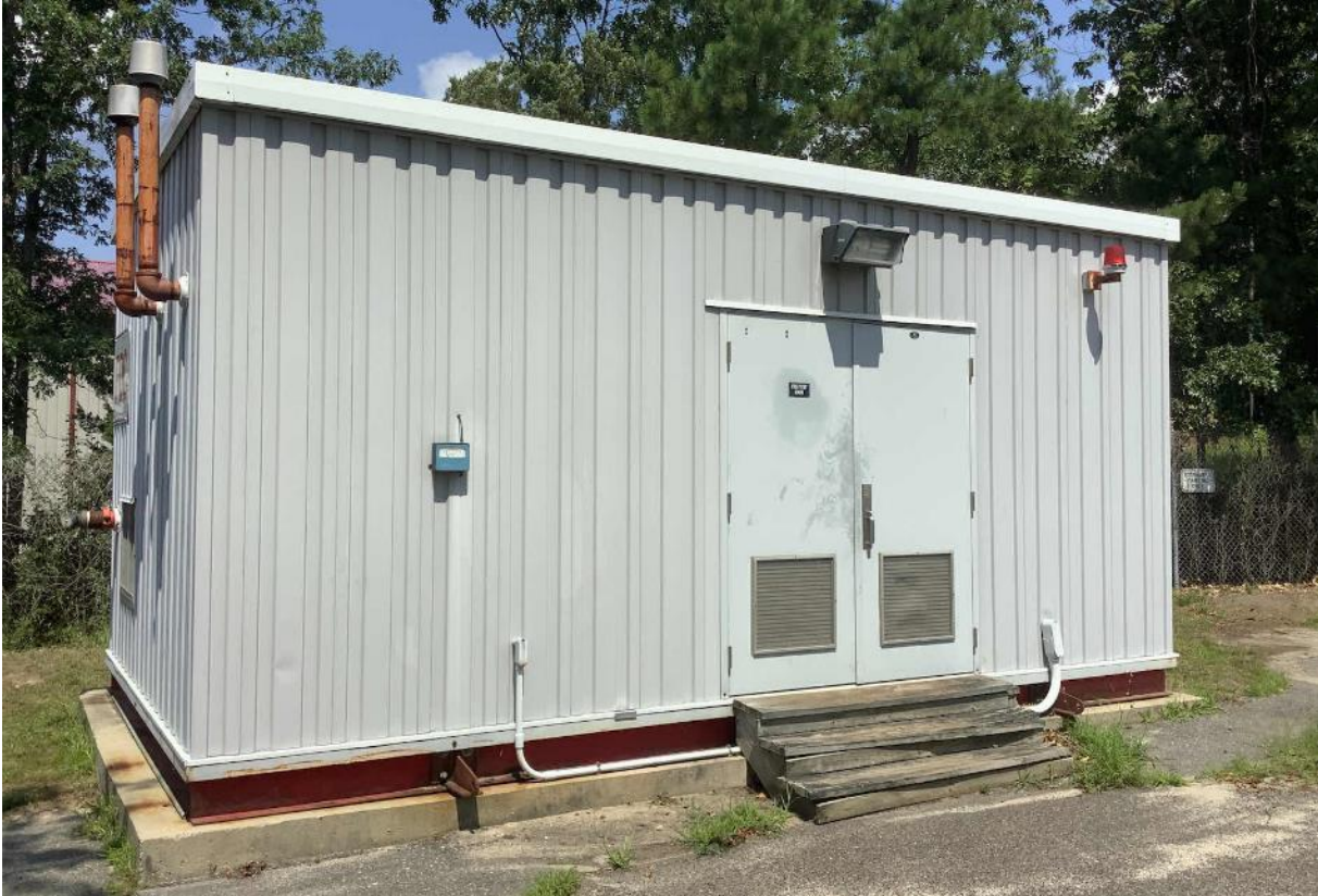
Fire Pump Building
