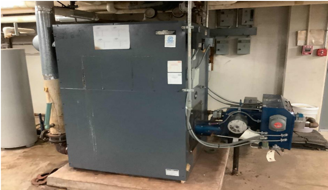
Hot Water Boiler
