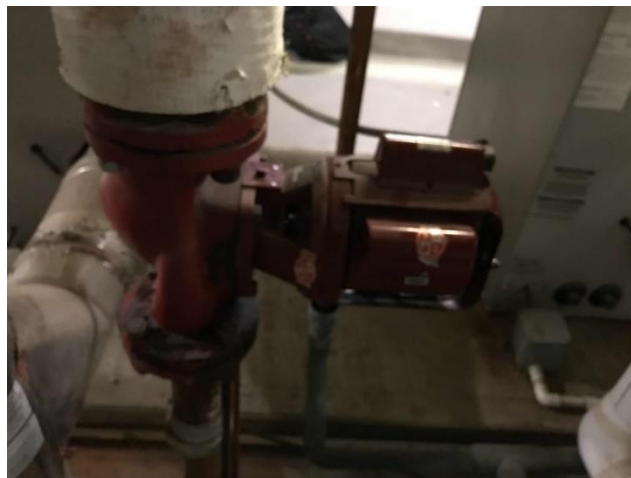
Heating Hot Water Pump
