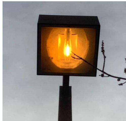
Exterior HPS Fixtures
