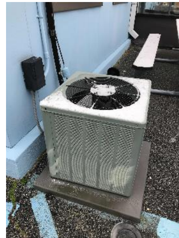
Condensing Unit for Split AC
