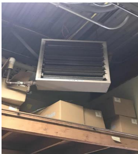
Typical Unit Heater
