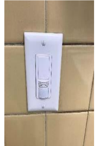
Occupancy Sensor in Restroom
