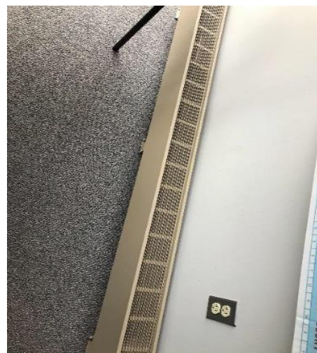
Electric Resistance Heater
