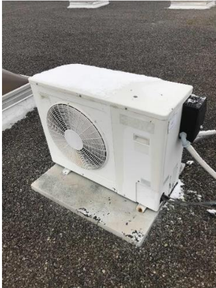
Mini-split Air Source Heat Pump
