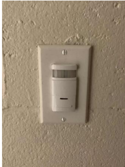
Wall Mounted Occupancy Sensor Switch
