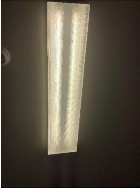
Surface Mounted Prismatic - T8 Linear Fluorescents
