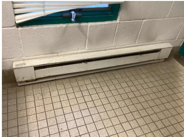
Baseboard Electric Resistance Radiator
