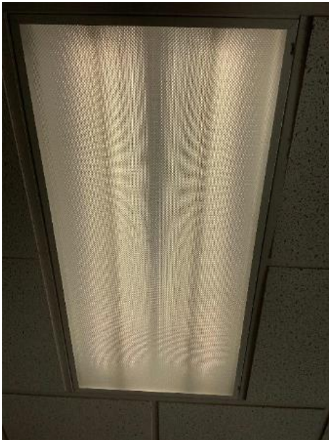
Recessed Prismatic Fixture
