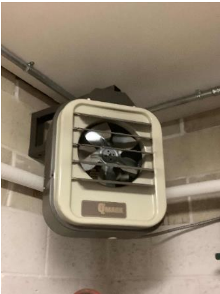
Suspended Electric Resistance Unit Heater
