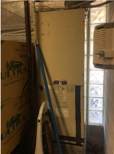
Mechanical Room AHU
