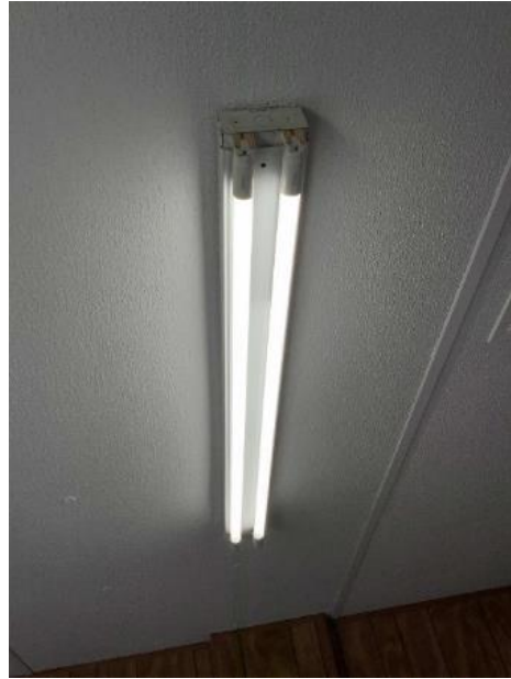
Surface Mounted Casing Removed – LED Equivalent
