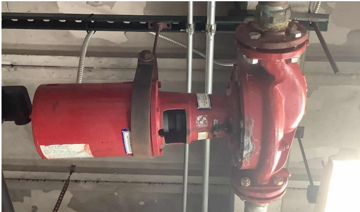
Heating Hot Water Pump
