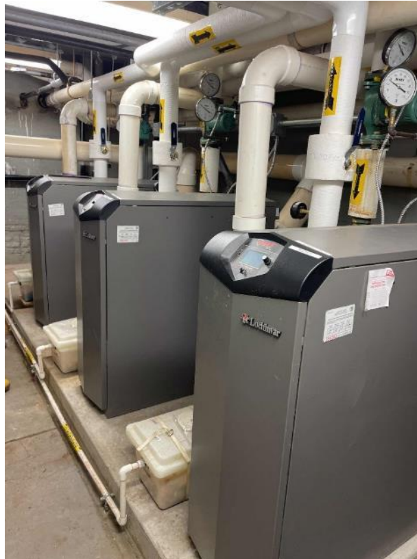
Hot Water Boiler Plant
