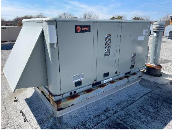
Central Distribution: Typical Package Unit
