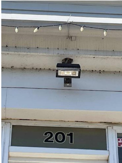
Stillwater Building: Exterior LED Fixture
