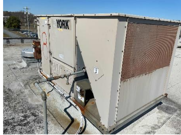
Central Distribution: Typical Package Unit
