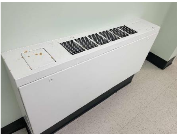
Central Distribution: Unit Heater
