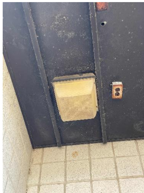
Central Distribution: Exterior MH Fixture
