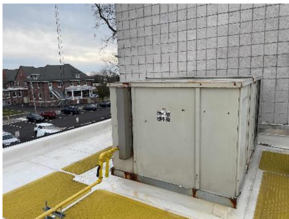
Stillwater Campus-Typical Package Unit
