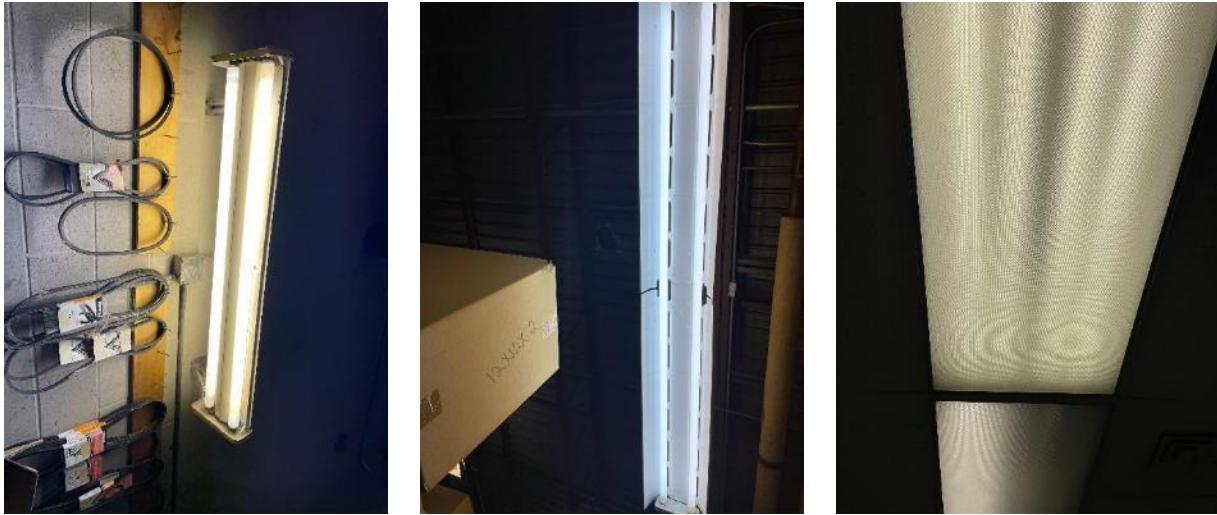
Central Distribution: Typical T8 Fluorescent Fixtures
