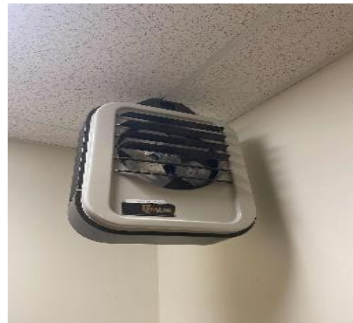
Central Distribution: Electric Resistance Heater
