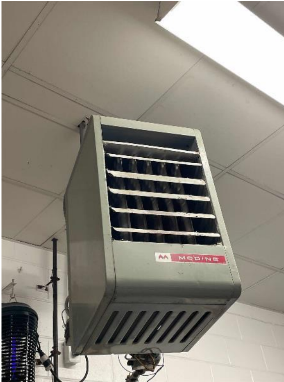
Central Distribution: Unit Heater
