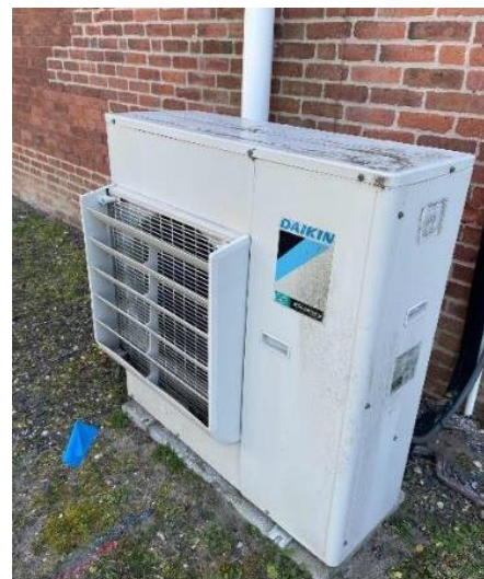
Stillwater Campus: Typical Split System Condensing Unit
