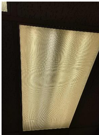
D Building: Typical T8 Fixtures
