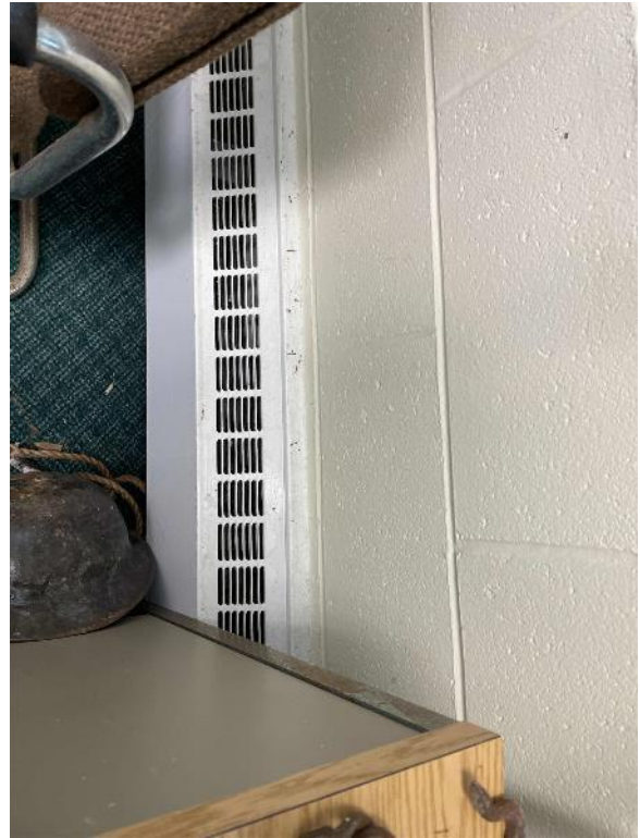
Central Distribution: Electric Resistance Heater
