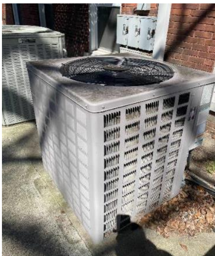
Stillwater Campus: Typical Split System Condensing Unit
