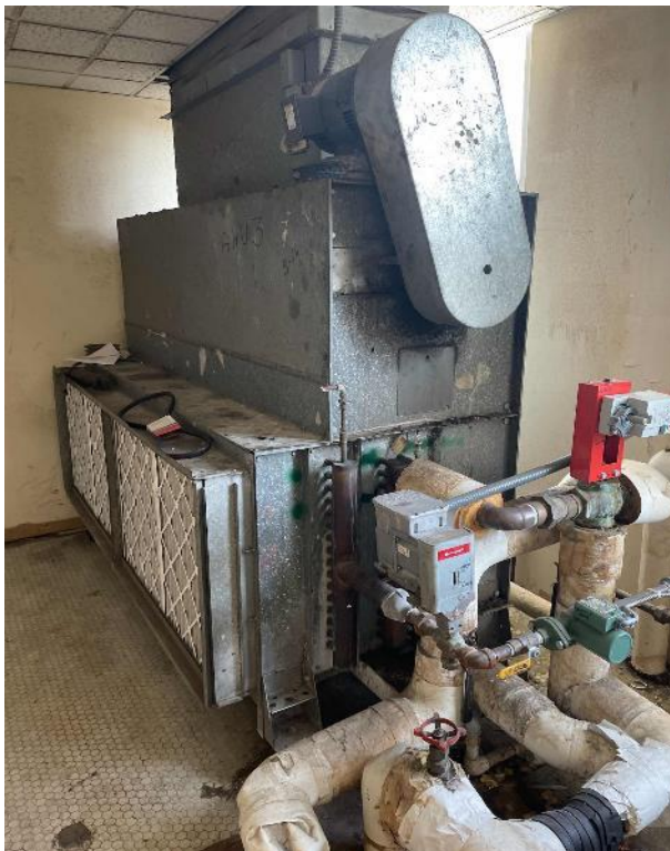
Stillwater Campus: Typical Air Handling Units
