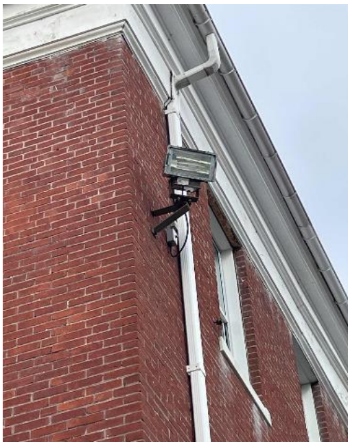
D Building Exterior MH Fixture
