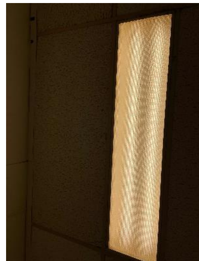
D Building: Typical T8 Fixtures
