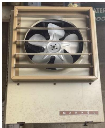
Electric Resistance Heater
