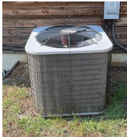
Split AC Condensing Unit
