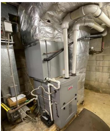
Propane Forced Hot Air Furnace
