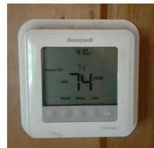
Programmable Thermostat
