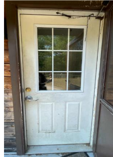
Fiberglass Facility Door with Glass Lite
