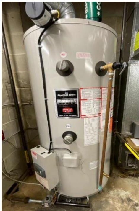
Propane-Fired DHW Tank
