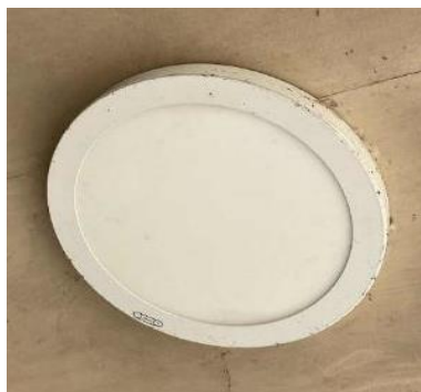
Exterior Surface Mounted LED Downlights
