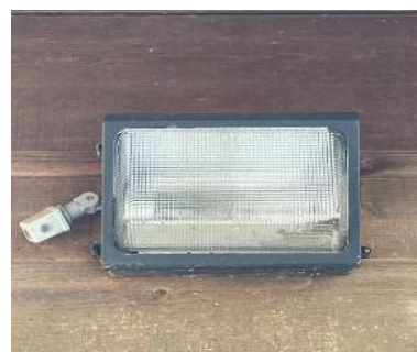
Exterior LED Wall Pack with Photocell
