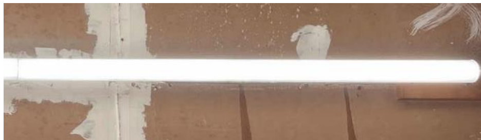
Maintenance Garage: 4-Foot LED Surface Mounted Fixture
