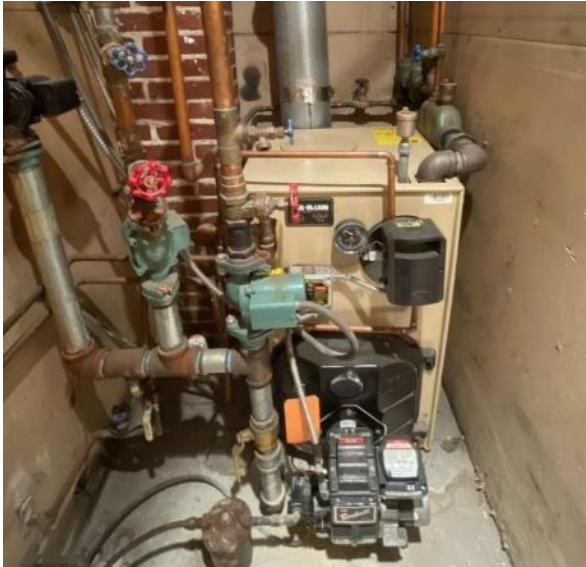
Maintenance Office Shop: Non-Condensing Boiler
