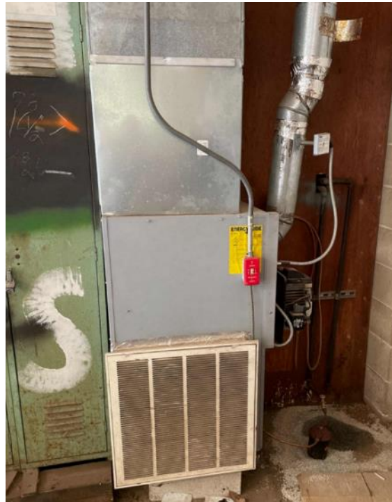
Maintenance Garage: Forced Air Furnace
