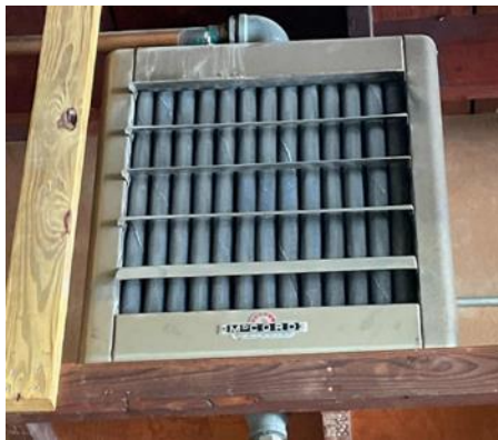
Maintenance Office Shop: Hydronic Unit Heater
