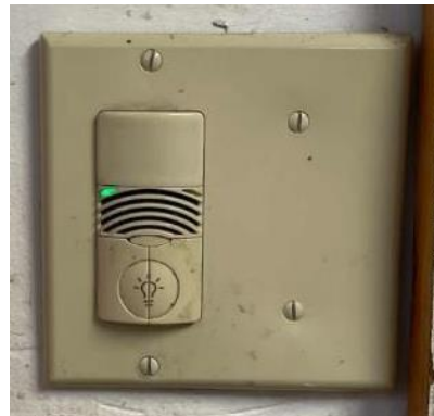
Wall Mounted Occupancy Sensor
