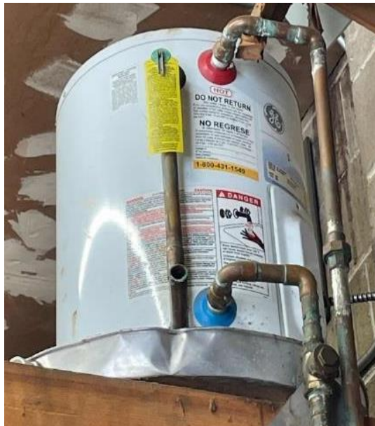
Maintenance Garage: DHW Tank
