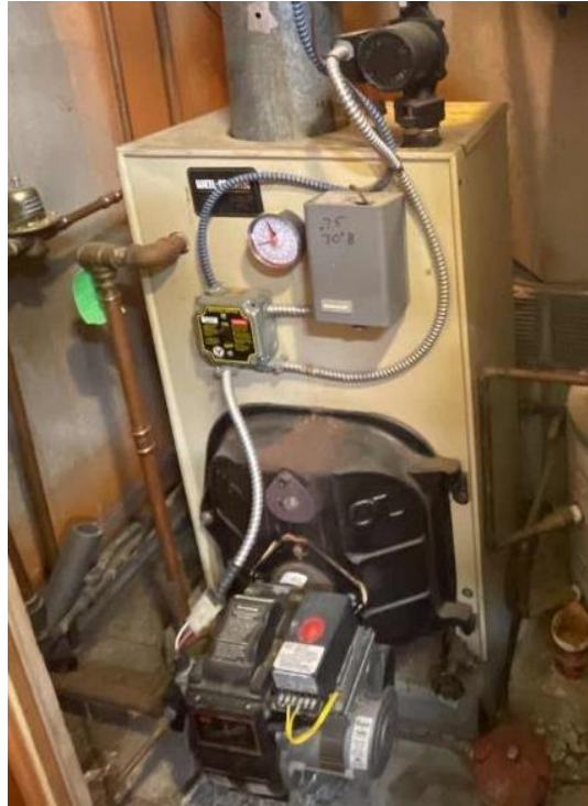
Interpretive Center: Non-Condensing HHW Boiler
