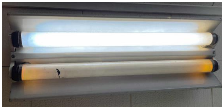
Interpretive Center: Surface Mounted T12 Lamps
