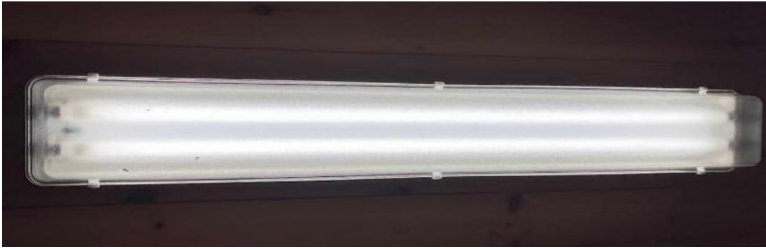
Interpretive Center: 4-Foot Linear Fluorescent T8 Lamps
