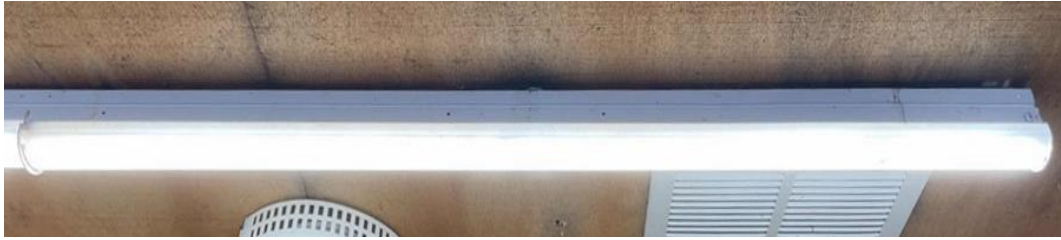
Meisle Campground Bathhouse: 4-Foot Linear LED Fixture
