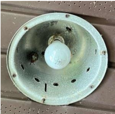
North Shore Bathhouse: Recessed Can A19 Incandescent Lamp
