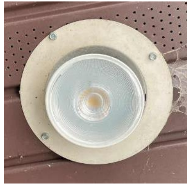
North Shore Bathhouse: Recessed Can PAR38 LED Lamp
