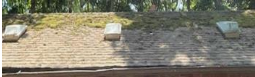
CCC Bathhouse: Roof with Moss
