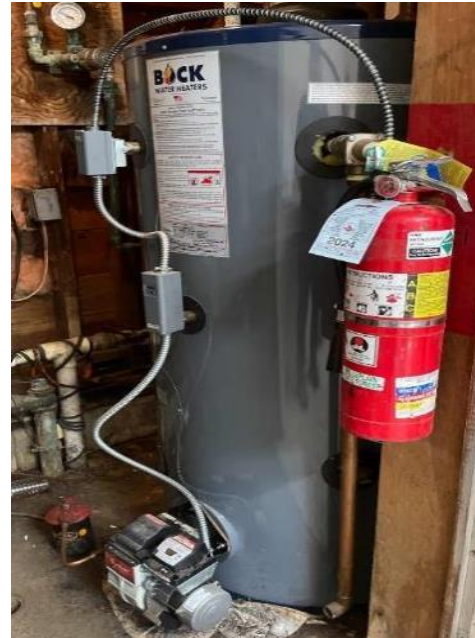
CCC Bathhouse DHW Tank
