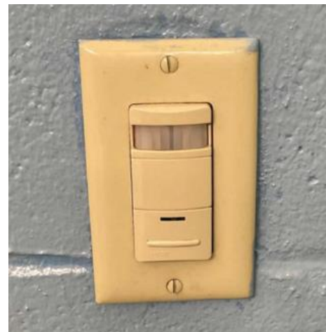
North Shore Bathhouse: Wall Mounted Occupancy Sensor
