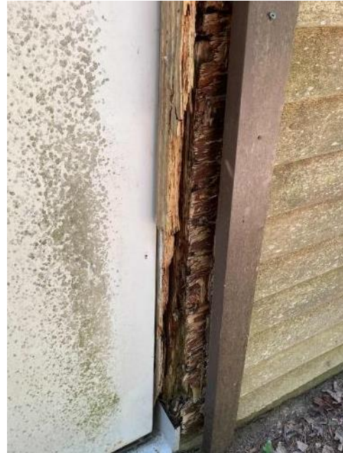
Meisle Campground Bathhouse: Poor Frame Condition
