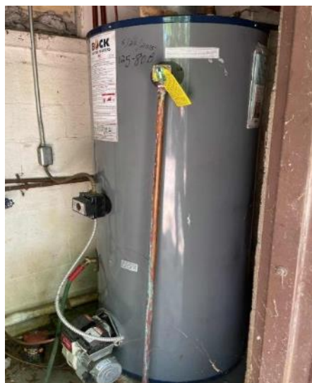
North Shore Bathhouse: DHW Tank
