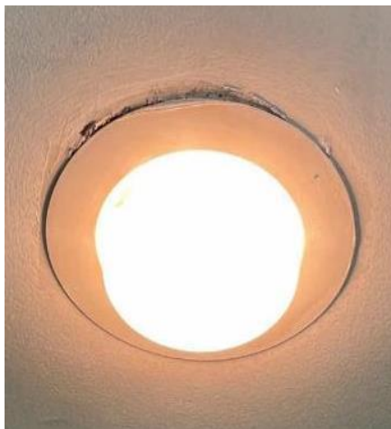
North Shore Bathhouse: Recessed Can CFL
