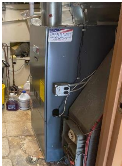
Oil-Fired Forced Hot Air Furnace
