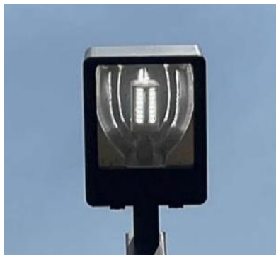
Pole Light LED Corn Bulb Retrofit
