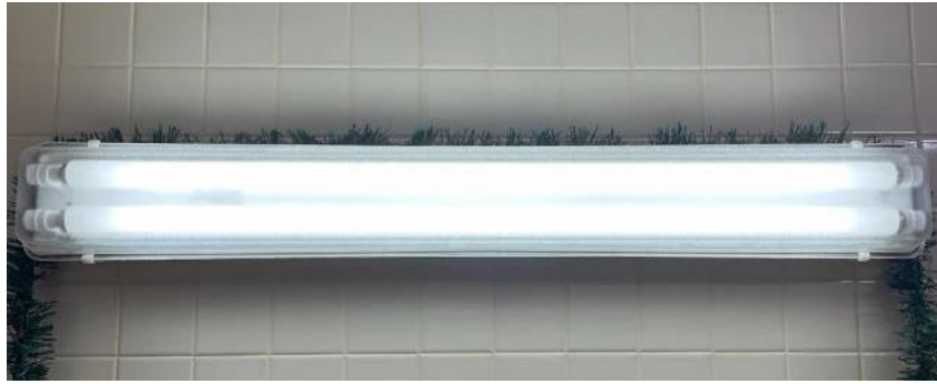
4-Foot T12 Linear Fluorescent Restroom Lighting
