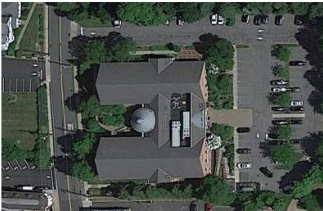
Aerial View of Facility
