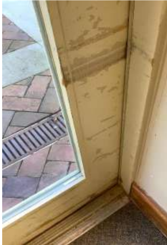
Wood Door Condition
