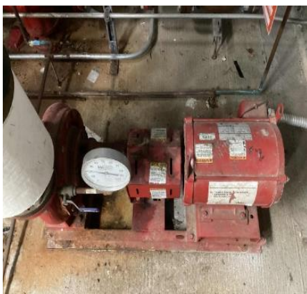
Heating Hot Water Pumps
