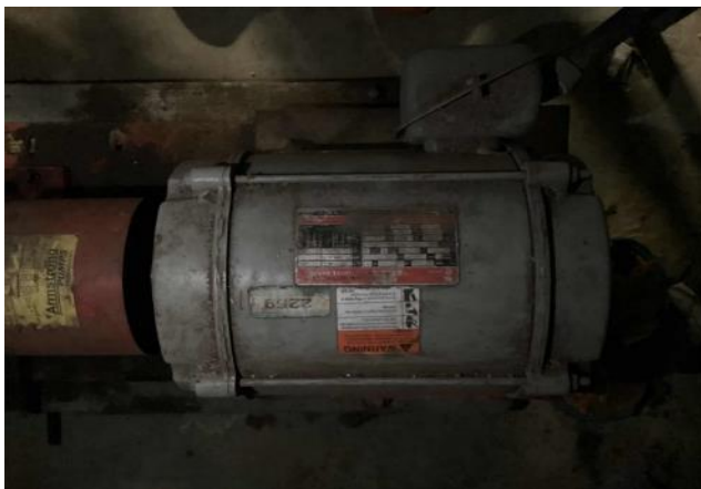
Heating Hot Water Pump
