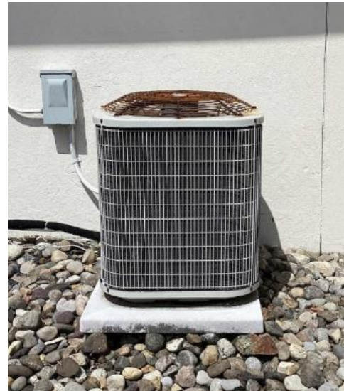
Exterior Condensing Units
