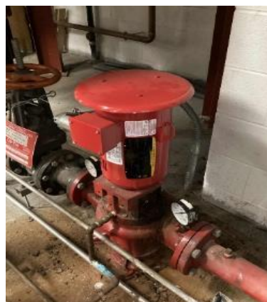
Heating Hot Water Pumps
