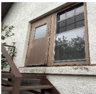
Second Floor Emergency Exit
