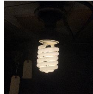
CFL in Basement Mechanical
