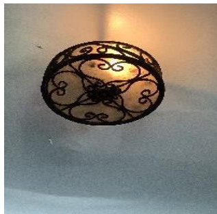
Corridor Ceiling Mounted Fixture
