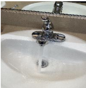
Restroom Sink 2.0 gpm
