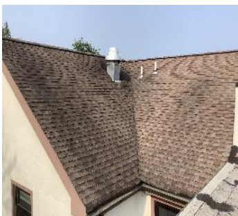
Pitched Roof with Asphalt Shingles
