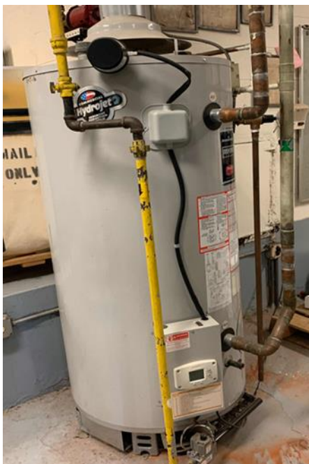
Domestic Storage Tank Water Heater
