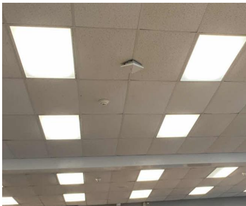
Linear T8 Fixtures and LED Exit Sign
