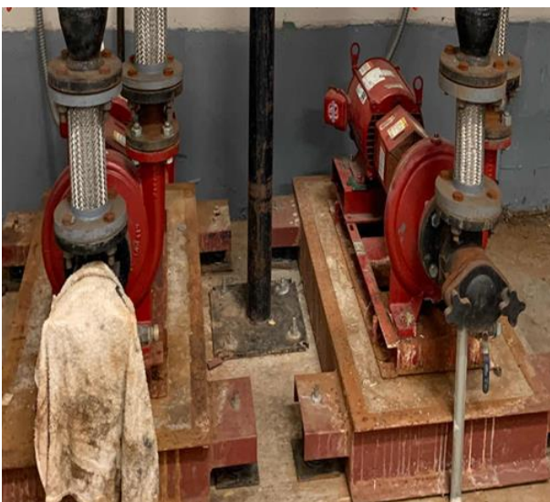
Heating Hot Water Pumps
