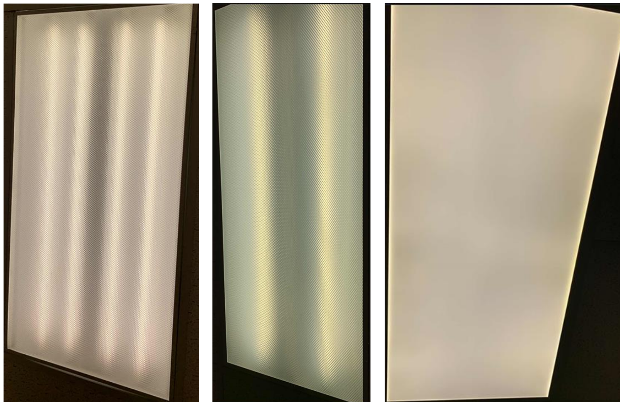
Linear T8 and 2x4 LED Panel
