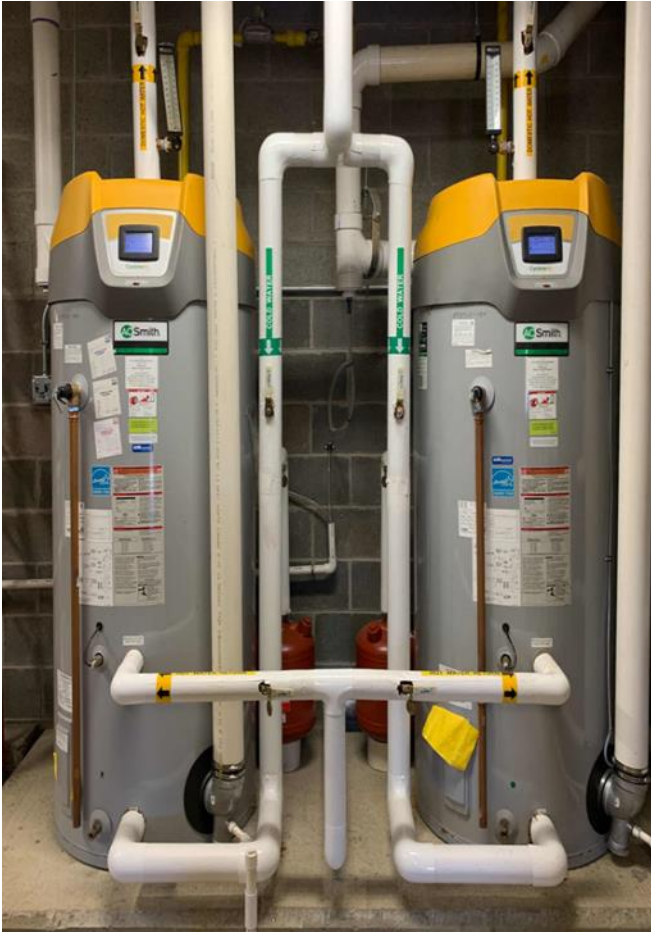
Domestic Hot Water Heaters and Circulating Pumps
