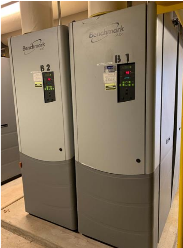
Condensing Boilers
