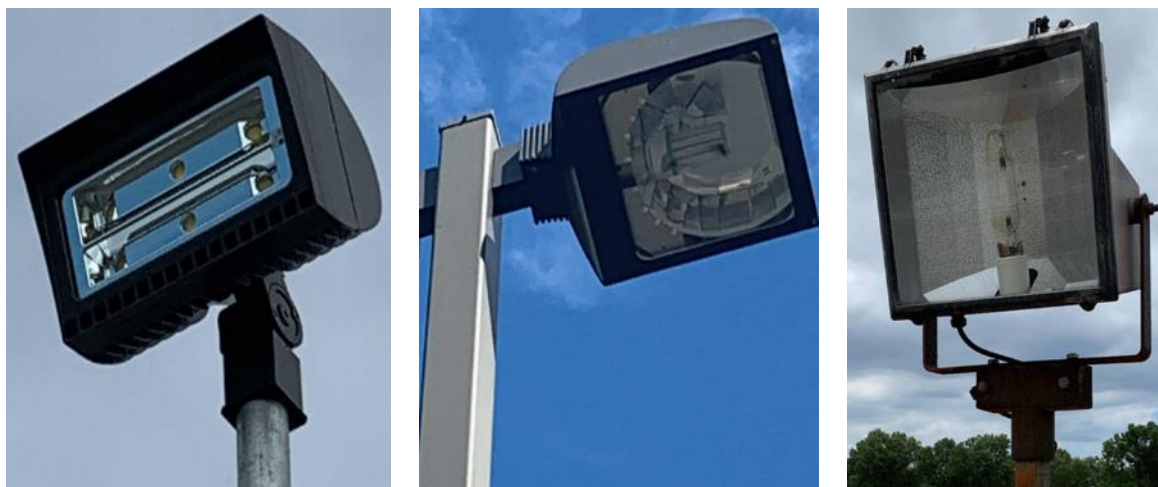
Pole Mounted LED Fixture, LED Corn Bulb, and Metal Halide Lamp
