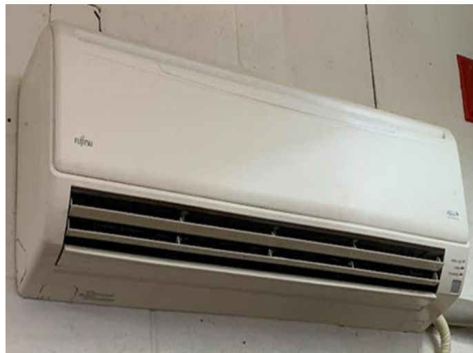
Split Air Source Heat Pump
