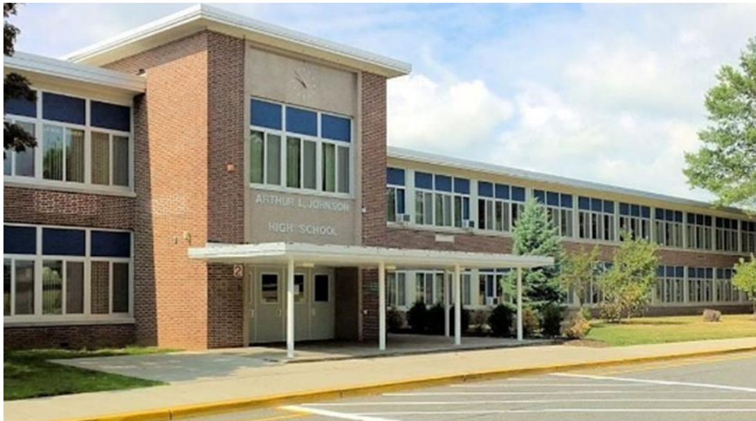
Front Building Walls
