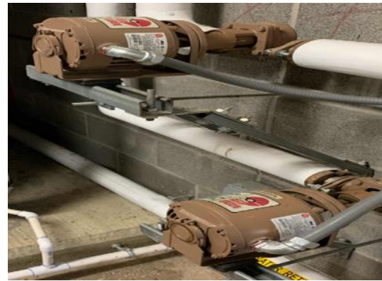
Domestic Hot Water Heaters and Circulating Pumps
