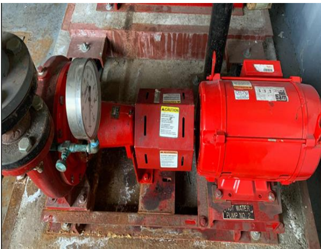
Heating Hot Water Pump
