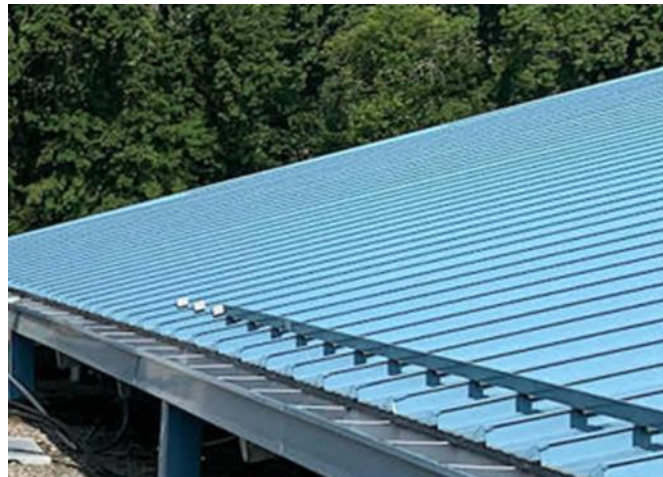
Flat Pebbles and Pitched Standing Seam Metal Roofs
