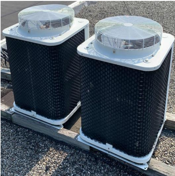
Condensing Unit - Split System ACs
