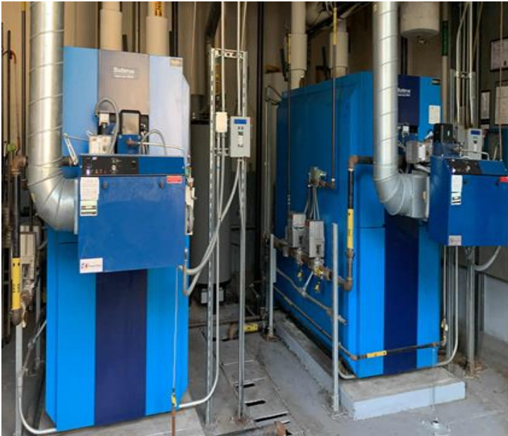
Non-Condensing Hot Water Boilers
