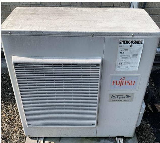
Split Air Source Heat Pump
