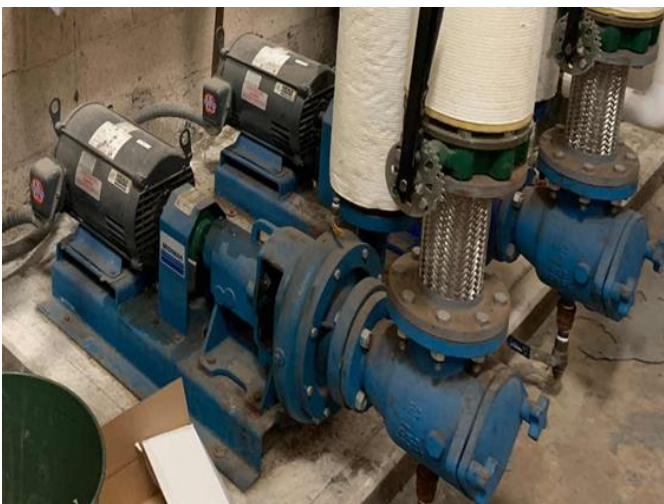
10 hp Variable Speed Hot Water Pumps
