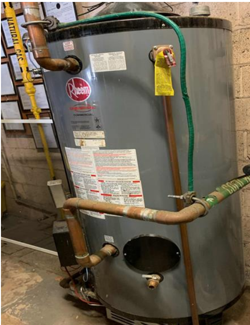
Gas-Fired Domestic Hot Water Heater
