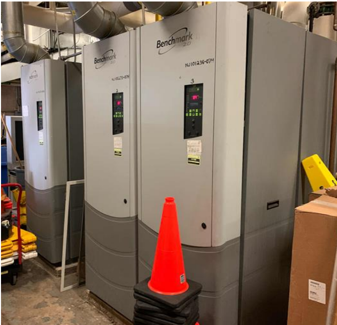
Aerco Condensing Boilers
