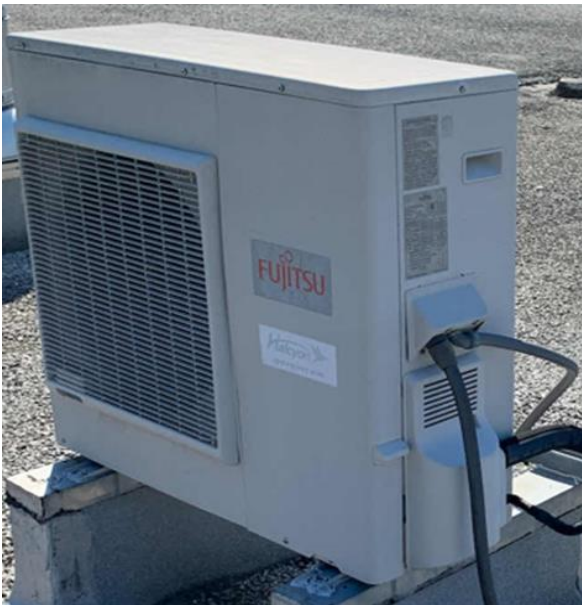
Split Air Source Heat Pump
