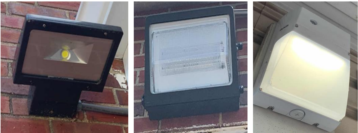
Wall Mounted LED and CFL Fixtures
