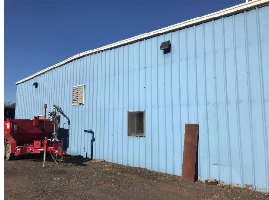
Side of Building
