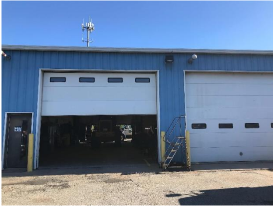
Front of Building
