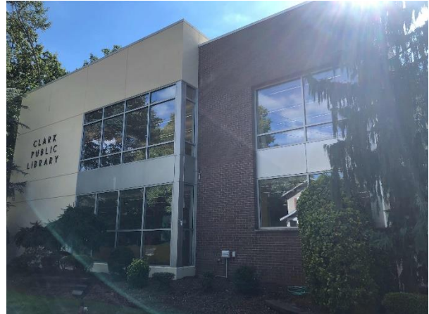
Side of Building
