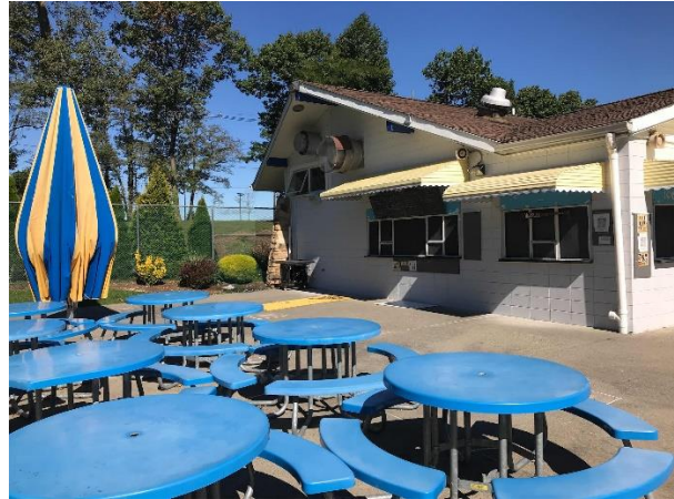
Side of the Building
